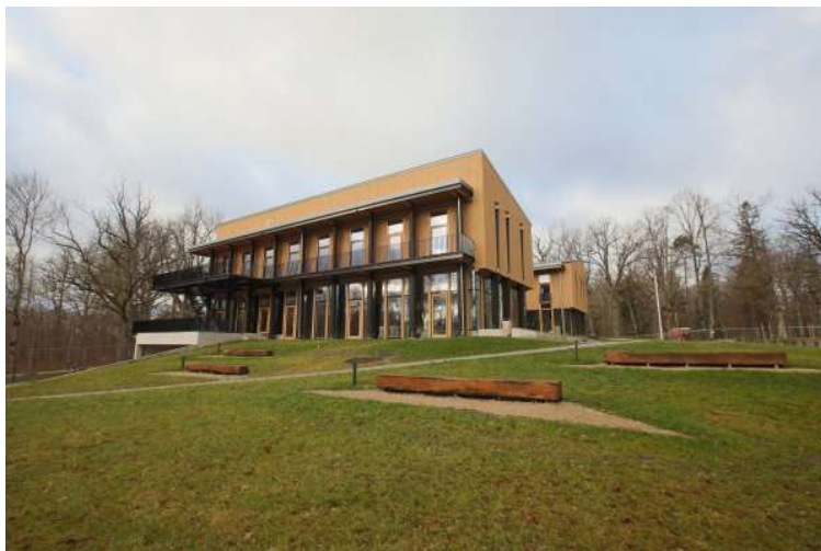
Fig. 3.2. Wooden building - 1st place for client center in Dundaga, Latvia, year 2016. Source: Latvia State Forests, 2017.
