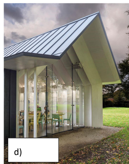
Fig. 3.15. Rievaulx Abbey Visitor Centre and Museum: a) Exterior view of the visitor centre (RIBA, 2017); b) Interior view of café (RIBA, 2017); c) white glulam arches (RIBA, 2017); d) Splayed glulam arches project beyond the glazed east gable (TRADA, 2019)
