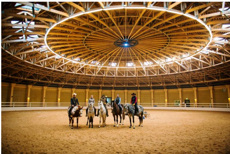
Fig. 3.11. The load bearing solid timber structure of the horse riding building (Makalius, 2018)
