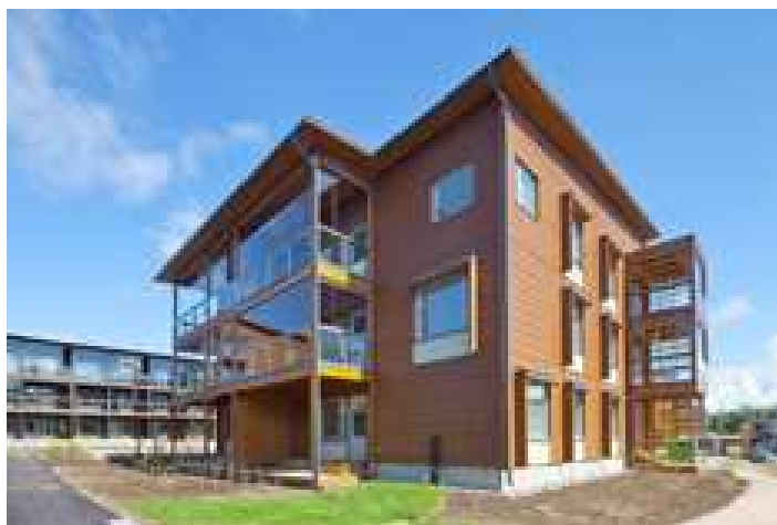
Fig. 3.13. An apartment building block in Latokartano, Viikki
