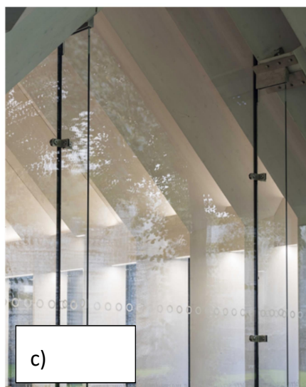
Fig. 3.15. Rievaulx Abbey Visitor Centre and Museum: a) Exterior view of the visitor centre (RIBA, 2017); b) Interior view of café (RIBA, 2017); c) white glulam arches (RIBA, 2017); d) Splayed glulam arches project beyond the glazed east gable (TRADA, 2019)
