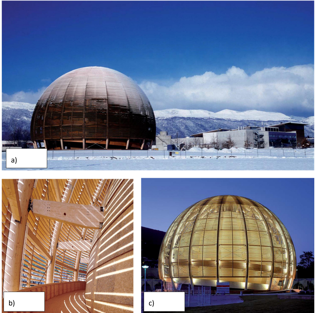
Fig.3.27. The Globe at CERN: a) A relocatable exhibition pavilion made entirely of wood; b) The interspace between outer and inner domes; c) The Globe at night
