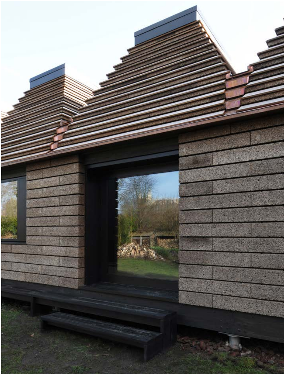
The walls and roof were fabricated from solid expanded cork blocks.
