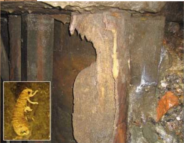
Marine-borer damage to a buried pile
