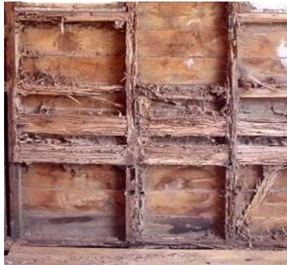
Termite damage
