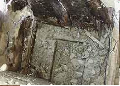
Marine-borer damage to a buried pile
